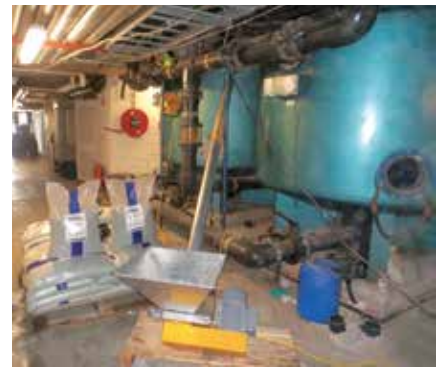
30 tonnes of Waterco EcoPure Glass Media replaced the sand filter media in five steel fabricated filters.
