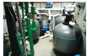
Four Micron SD750 fibreglass wound filters, with two high head Hydrostorm plus 200 pumps, and two MultiCyclone centrifugal pre-filters.
