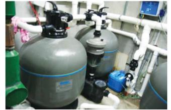
Each Hydrostorm plus 200 pump was plumbed to one MultiCyclone filter and the flow was split between two Micron SD750 filters.
