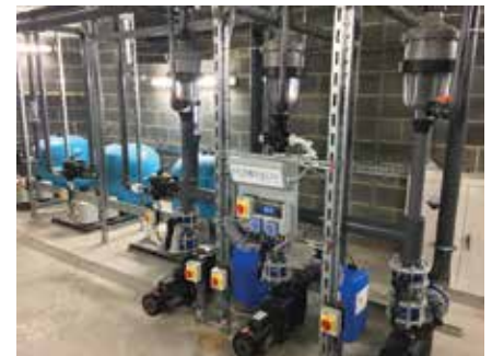
Waterco’s Hydroxypure chlorine-free sanitisation system was chosen for the two naturally treated lagoons.
