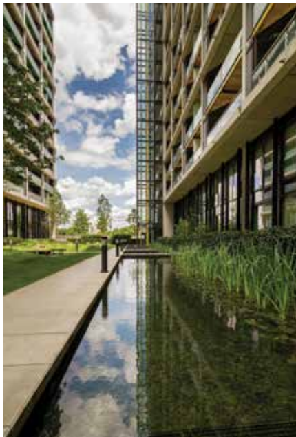
Riverlight consists of 806 apartments located in the heart of the new Nine Elms development on London's South Bank.
