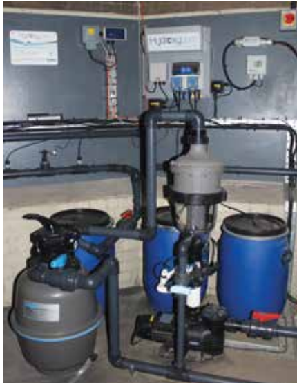
Waterco's T450 sand filter, Aquamite pump and Hydroxypure system work together to run the restaurant's prominent water feature.
