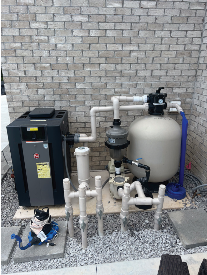
MultiCyclone prevents up to 80 percent of the filter's incoming dirt load, easing the workload of the pool's filter media.
